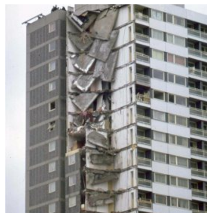
Large concrete panel buildings, a popular form of post-war construction, fell out of favour after the Ronan Point disaster in east London in 1968, when a gas explosion caused the panels to slip and collapse, killing four people. (Photo source: Wikipedia)
